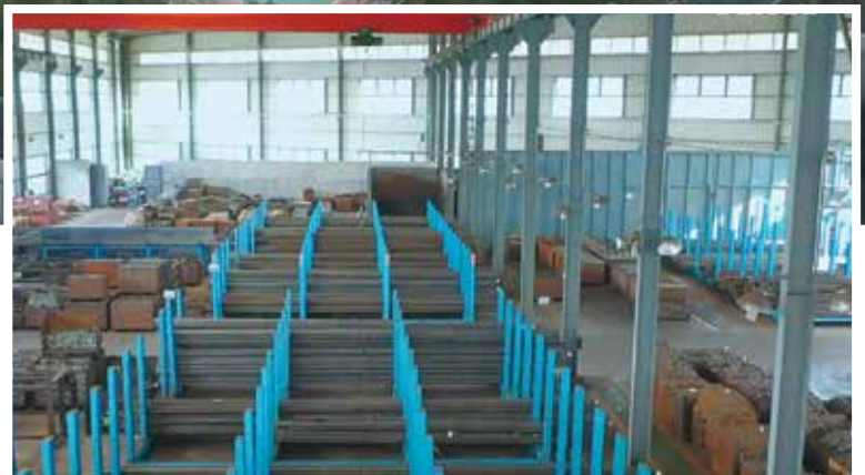
Raw Materials Plant
